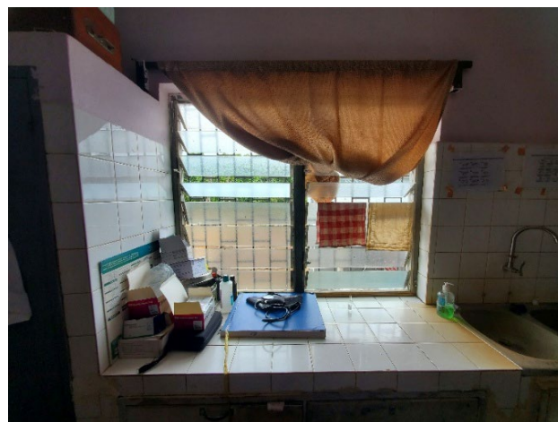
Figure 30: USP Sagbiebou: louvered windows with glass and wooden frames used for room ventilation.
