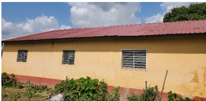
Figure 11: Aluminum tray roof – USP Tchalo
