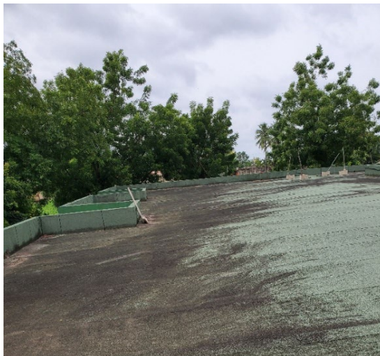
Figure 36: USP Atchangbade: waterproofing of the slab is locally deteriorated due to continuous presence of water on the slab, with no clear separation to ensure patient privacy, and a lack of effective drainage
