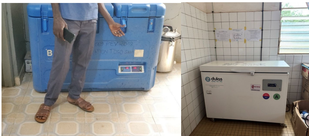
Figure 39: Cold chain: (a) USP Tchalo, functional; (b) USP Tindjassi, solar direct drive.
