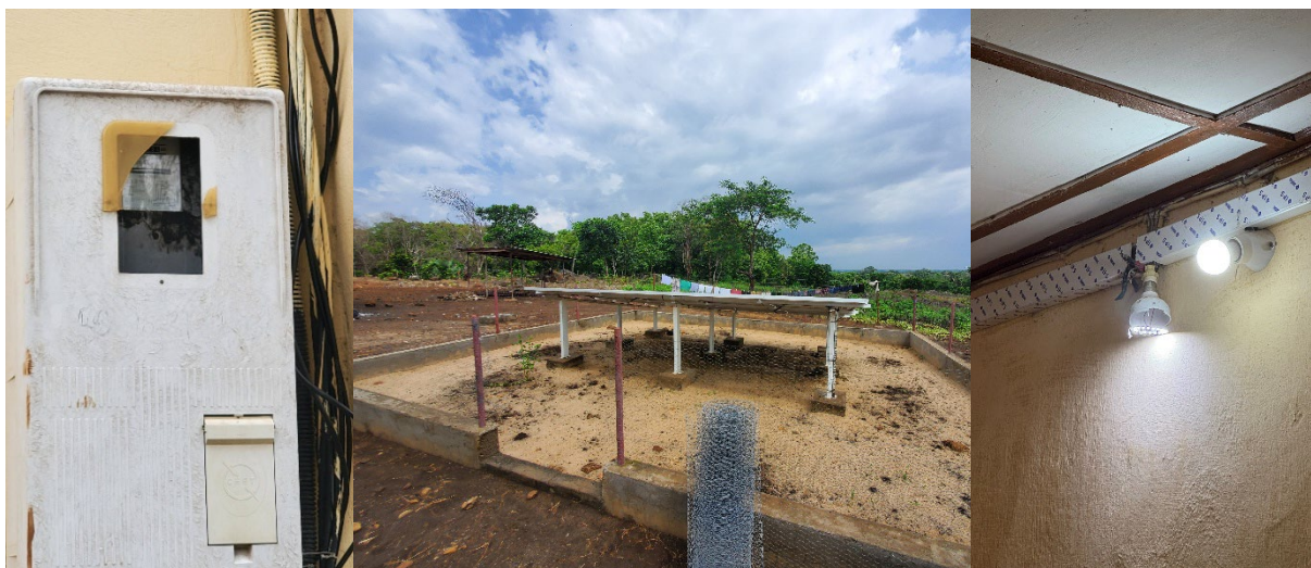
Figure 38: Sources of electrical energy in the USPs – (a) USP Atchangbade, CMS powered by the CEET network; (b) USP Kaza, centre fully powered by solar energy; (c) USP Tenega, mixed solar and CEET installation
