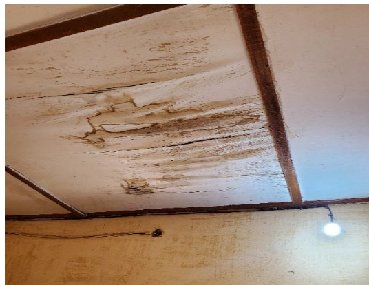
Figure 37: USP Tenega: roof in an advanced state of deterioration due to water infiltration from the roof
