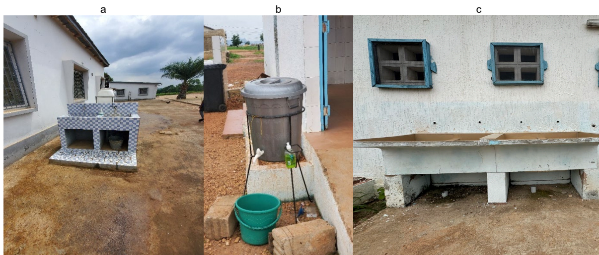
Figure 16: Handwashing systems (from left to right): (a) USP Kaza – fixed, connected system; (b) non-connected centre – makeshift facility; (c) outdoor sink – non-functional
