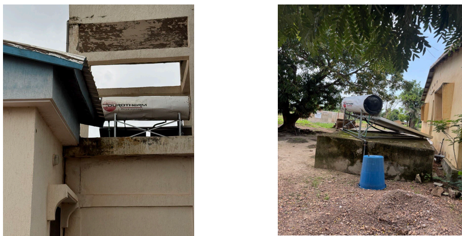
Figure 40: Solar water heater installations: (a) USP Sagbiebou – non-functional system installed under a slab, limiting sunlight exposure; (b) system installed on an external slab with exposed collectors, 2025
