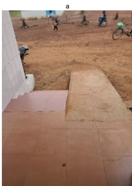
Figure 20: Accessibility of infrastructure (left to right): (a) USP Dakpankpergou – entrance ramp for persons with reduced mobility (PRM) without handrails; (b) USP Siou – entrance ramp for PRM equipped with handrails, 2025
