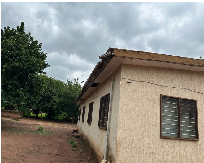
Figure 34: USP Tindjassi – existing rainwater drainage system but completely deteriorated and non-functional
