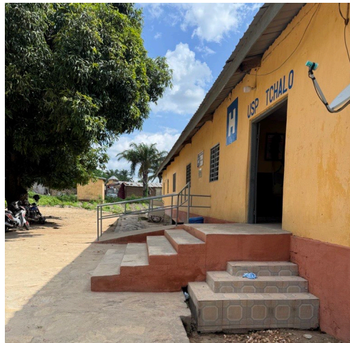
Figure 35: USP Tchalo – absence of a rainwater collection and drainage system at the building entrance
