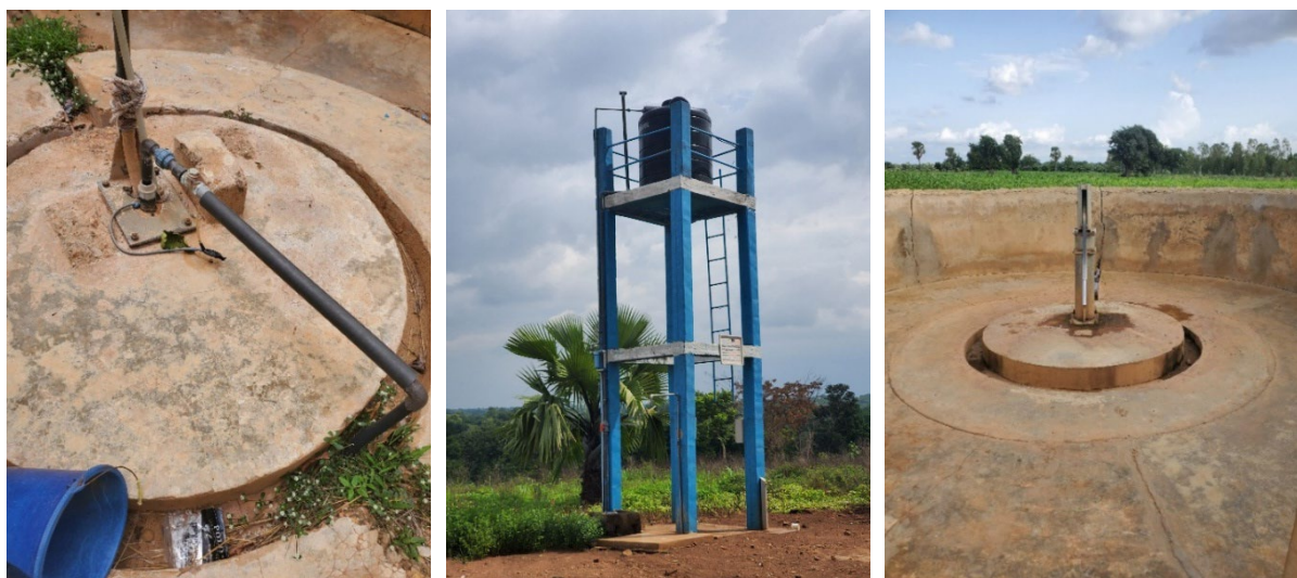
Figure 14: Water supply in three USPs: Sagbiebou – borehole with submersible pump on the left; Kaza – water tower in the centre; Dakpankpergou – manual borehole on the right
