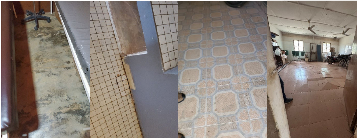
Figure 28: Floor coverings in the USP (from left to right): (a) USP Namare – smooth screed; (b) USP Kaza – floor tiles and waiting area bench, tiles detached; (c) USP Tchalo – floor tiles; (d) Room non-functional due to broken tiles
