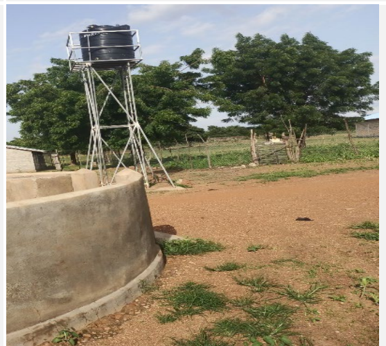
Elevated tank powered by a solar pump to allow gravity flow at the terminals
