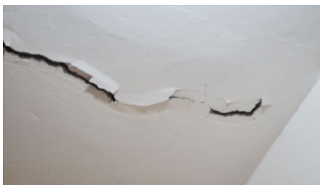
Figure 26: USP Atchangbade: Structural cracks in the slab
