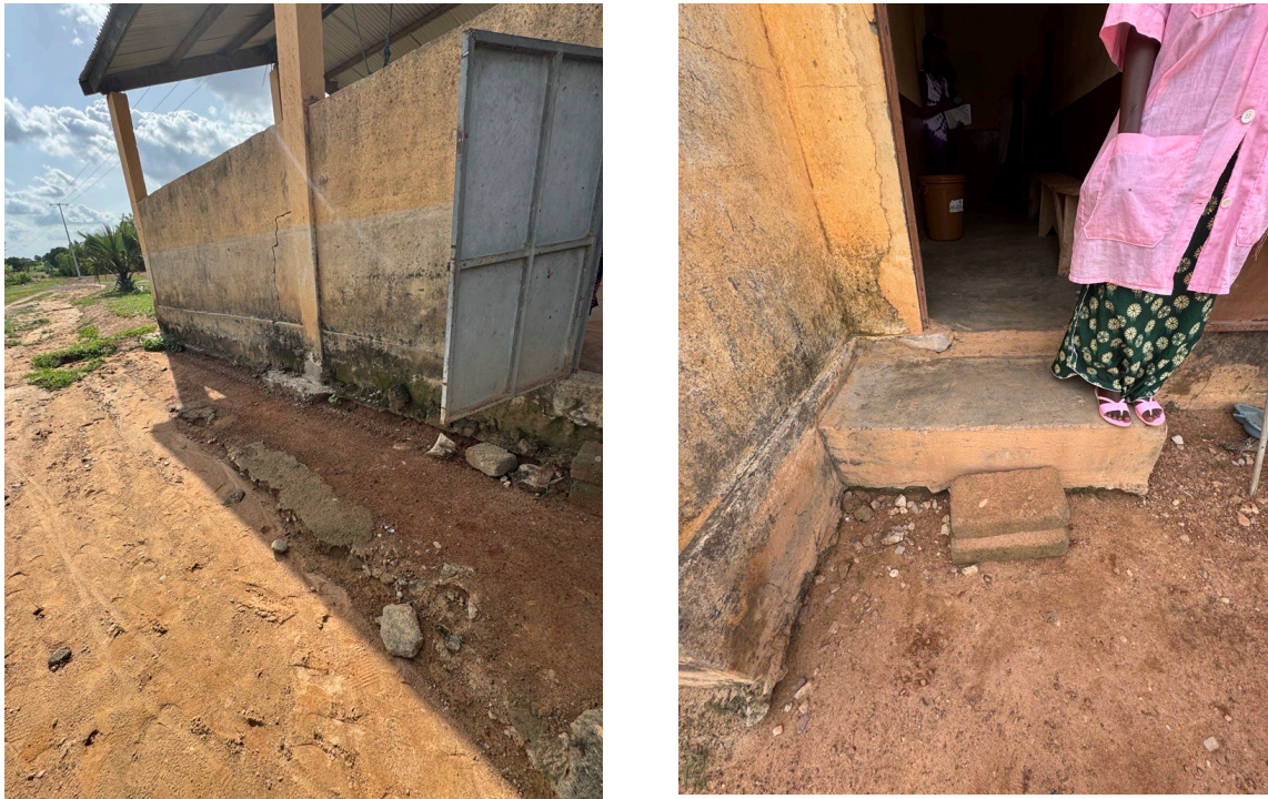
Figure 7: Effects of erosion on health infrastructure – case of the Namare USP, Savanes region
