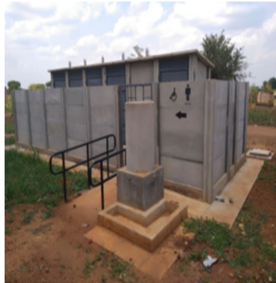
Figure 45: Prefabricated model of the walls of the concrete sanitary facilities
