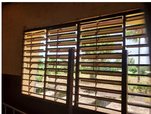
Figure 31: Louvered windows for room ventilation: (a) USP Tchalo – louvered windows with glass and wooden frames; (b) USP Tenega – metal louvered windows
