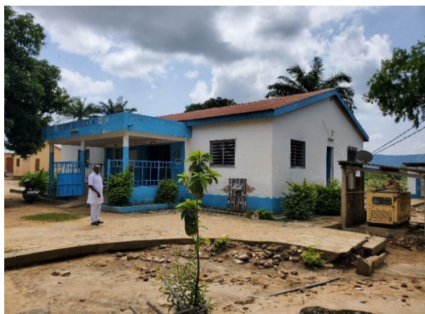
Figure 32: USP Tchalo: pitched roof with corrugated metal covering the general medicine building
